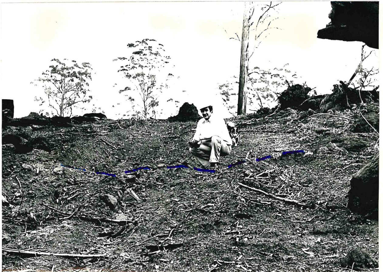
Plate 3. An erosion barrier on the snig track on the eastern end of the pinch illustrated on plate 1 of the S.W.F.D.F. Report. The course of the cross drain is outlined in the centre of the picture. Careful attention has been given to the question of erosion caused by snig tracks.
