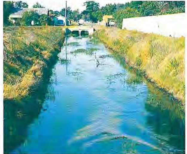
Plate 19 The Bayswater Main Drain
