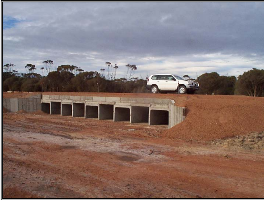
Culverts Under Pingrup – Newdegate Road
