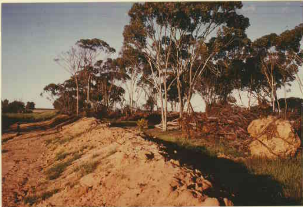
Freshly constructed drainage ridges on reserve. Note fallen timber.
