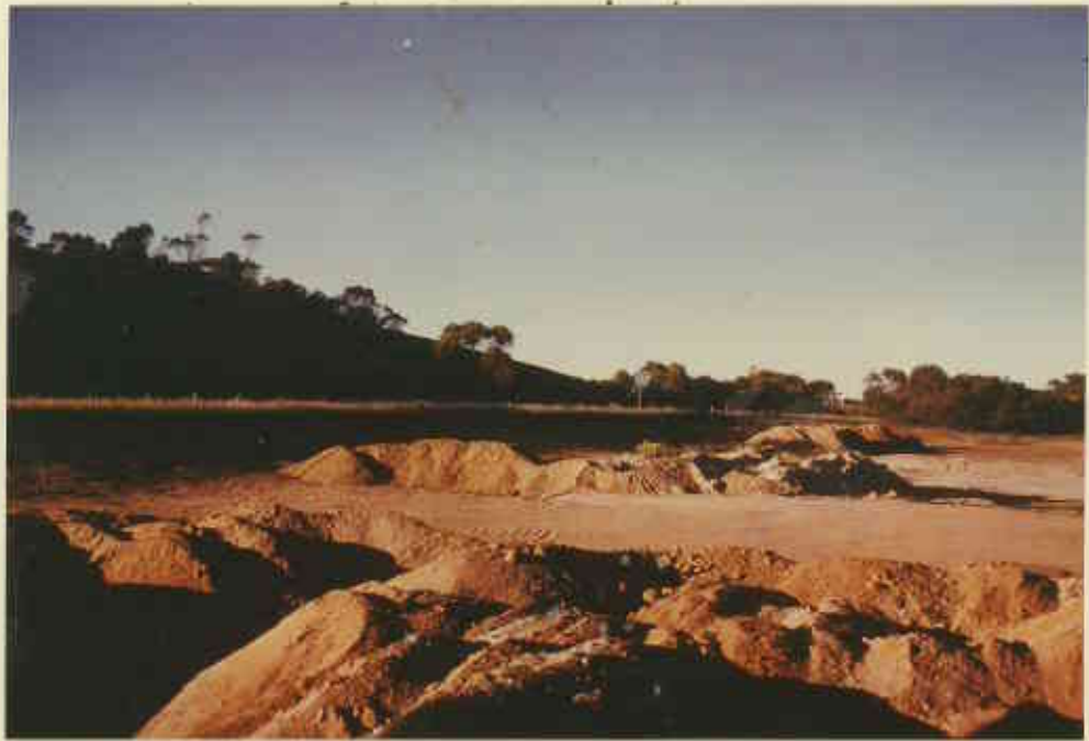
Earth excavations at base of Kwolyin Rock
