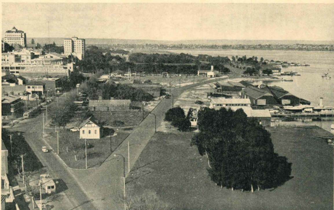
PERTH RIVER FRONT Showing the premises of boat builders and lightering com- panies, the eventual removal of which is intended
