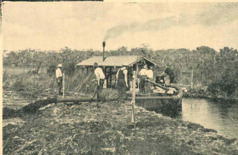
Dredging the stream bed to reclaim swampy banks
