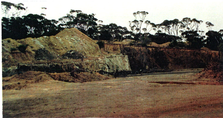
Plate 24: Open cut excavation of the vermiculite mine in the Young River corridor.
