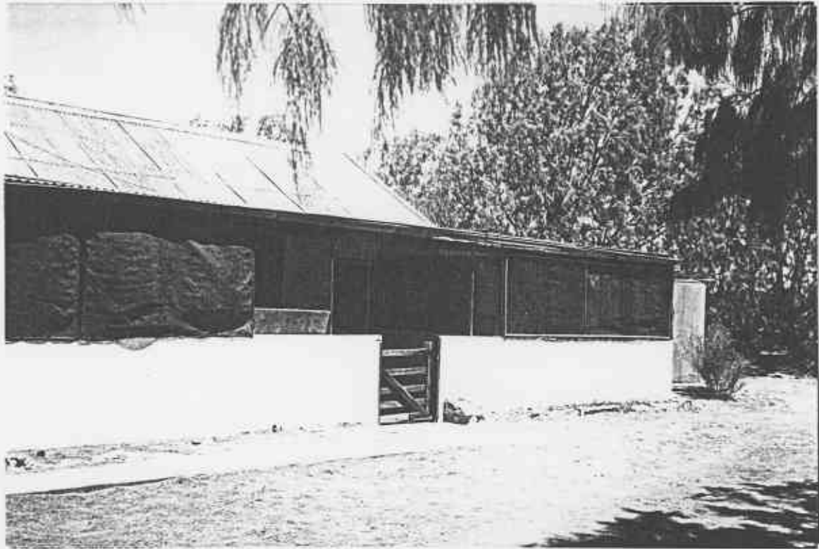
10.1.8 The entrance gate leading to Verandah 1. The two wooden framed glass louvre windows lead to Bedroom 1.
