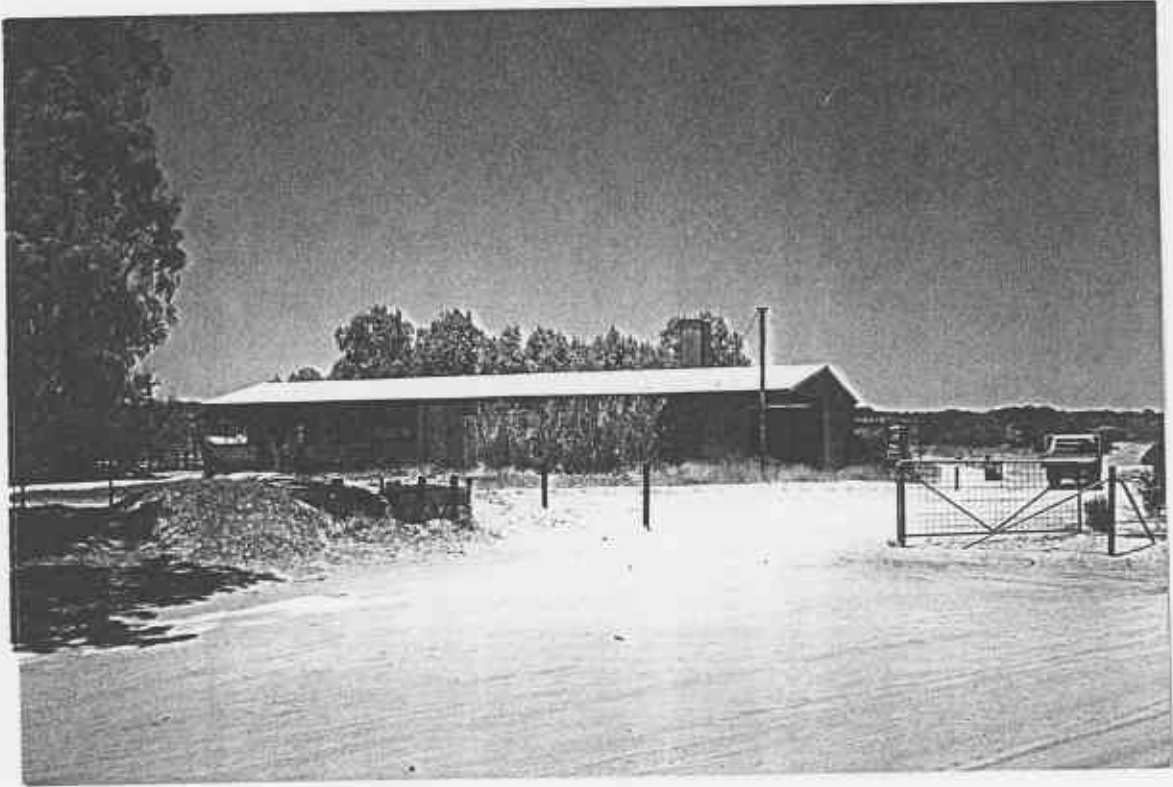
10.2.19 View of the Shearing Shed looking south.
