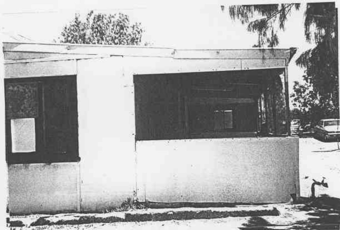
10.1.5 View of Verandah 1, looking north. Note the shell-cement blocks at the bottom of the photograph.
