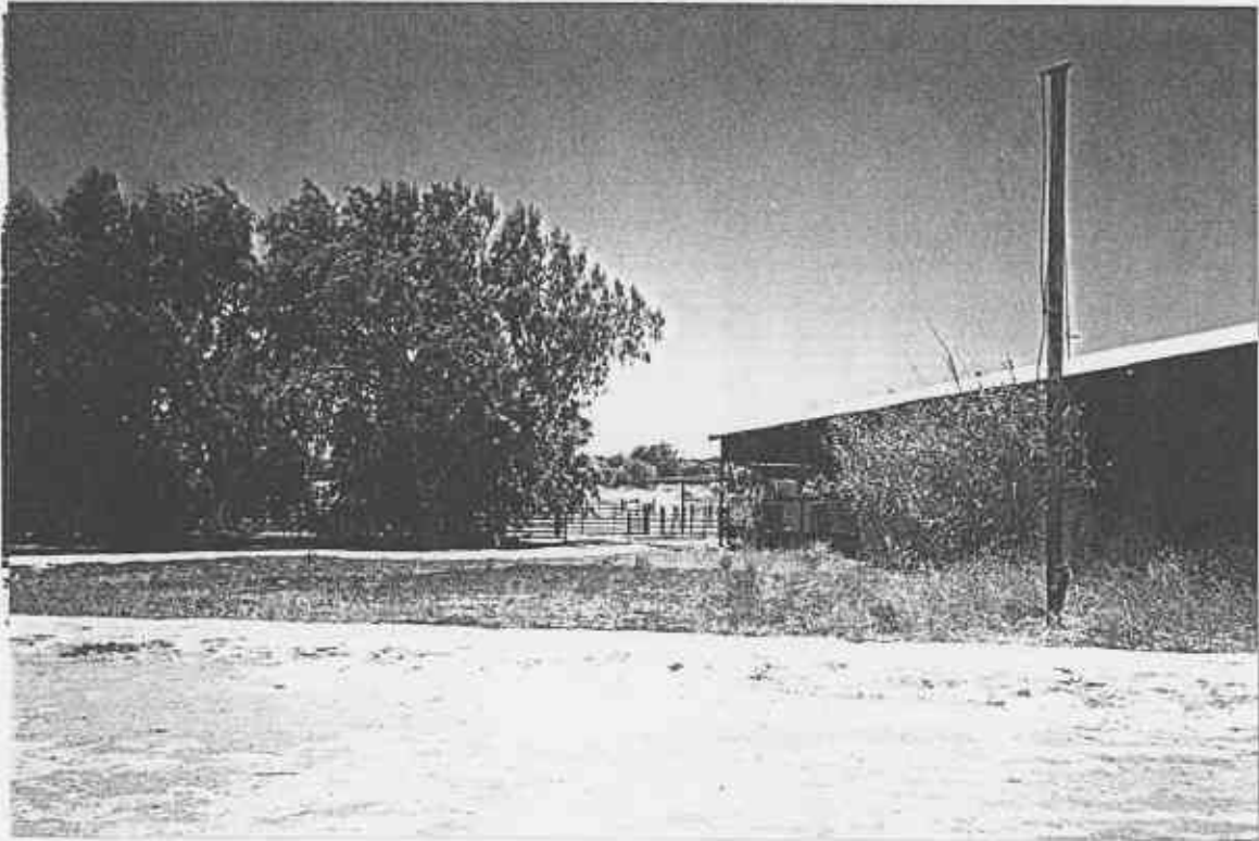
10.2.23 The sheep yards are constructed of 1" water pipe.
