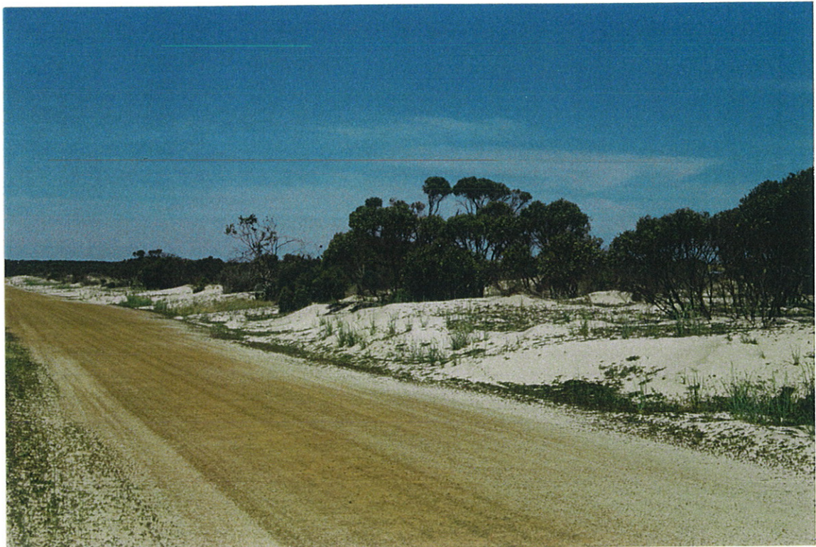
Photo 14. Severe sand blow across Fitzgerald Road
