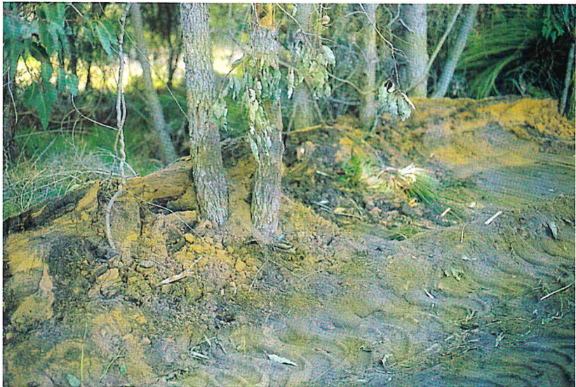
Poor location of stockpiles (Photo by David Lamont)
