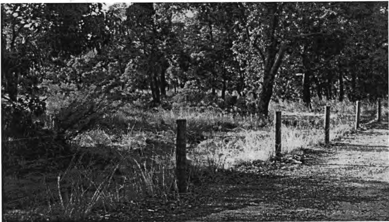
Preferred fencing style for Talbot Road Bushland – pine posts with ringlock fencing and a plain top wire
