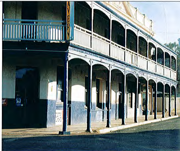
Buildings, roads, rail and water facilities are all at risk from salinity. Photo: Department of Conservation and Land Management
