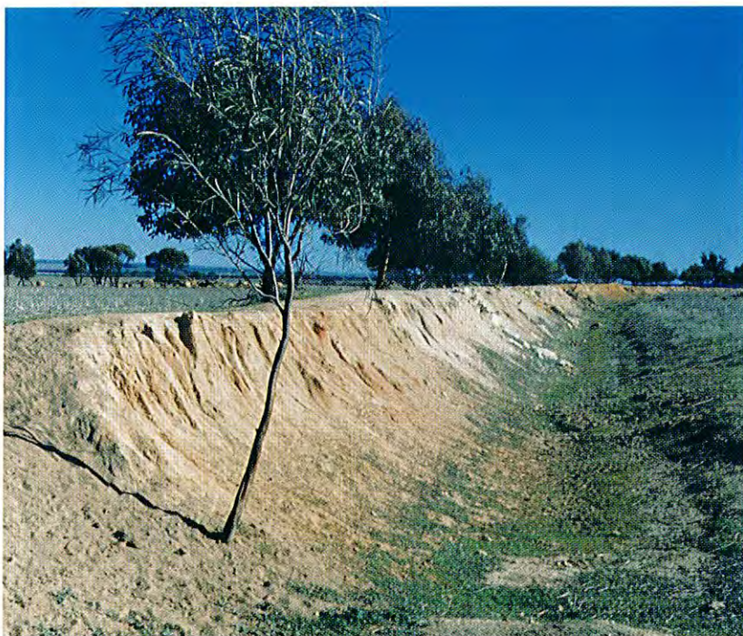
Contour bank to manage surface water. Photo: Landcare Vision
