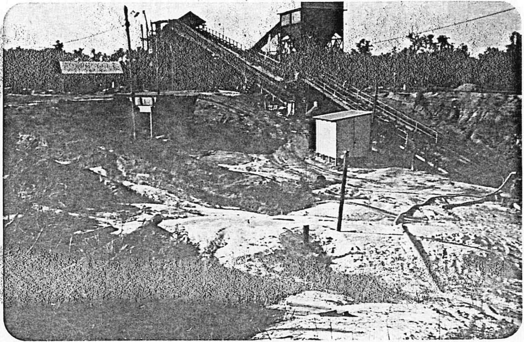
Centaur underground mine headquarters showing coal conveyer to hoppers at railway siding. Tunnel entrance is further to right. Mine closed 1957 but installations appear to be intact.
