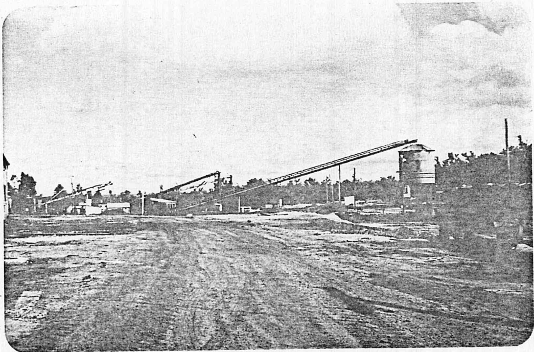
Western 2 underground mine headquarters showing coal conveyers from the mine to hoppers at rail head and coal heaps.
