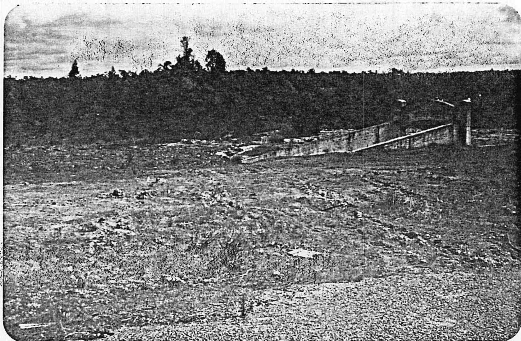
Stockton underground mine portal = tunnel entrance in cleared area at mine H.Q. In background is eucalypt planting P76? and regeneration since mine closed in 1957. In foreground eucalypts planted P82 in ripped lines.
