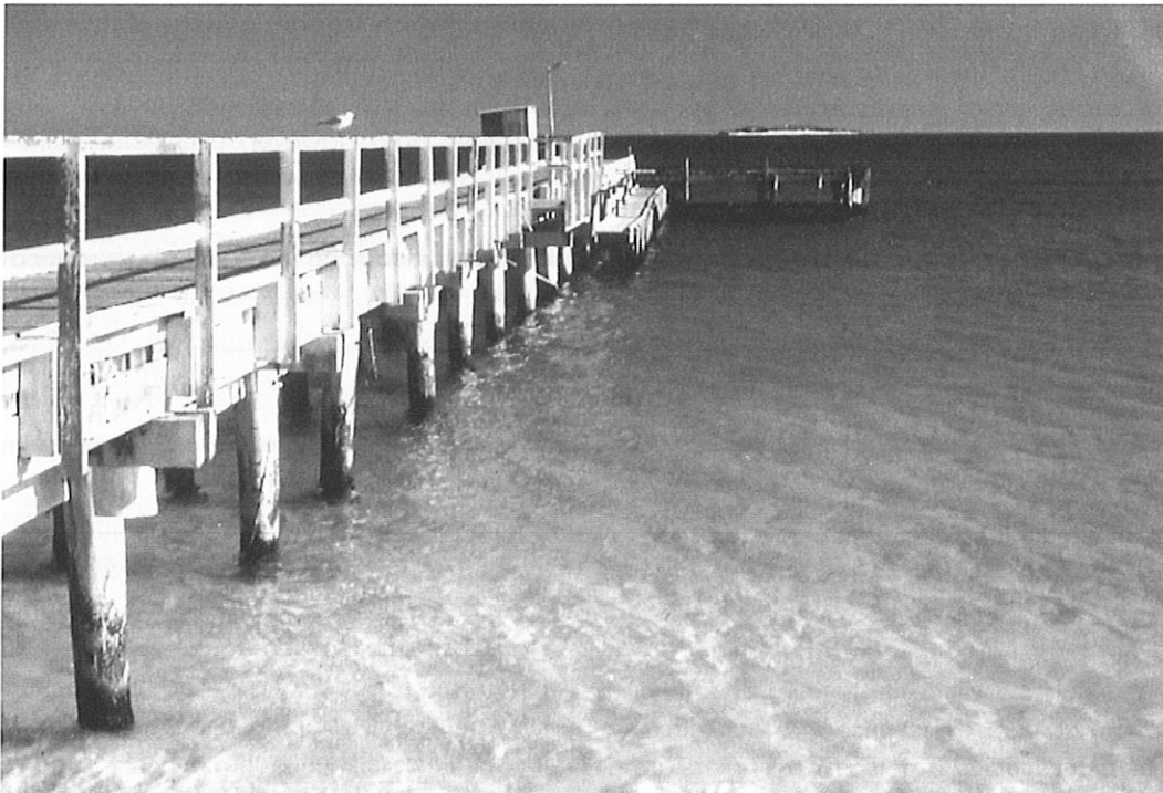
Jurien jetty provides boating facilities to the public.
