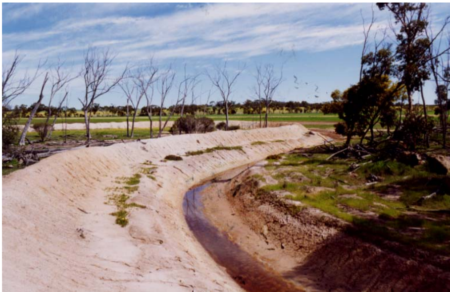
A shallow drain (Tammin)
