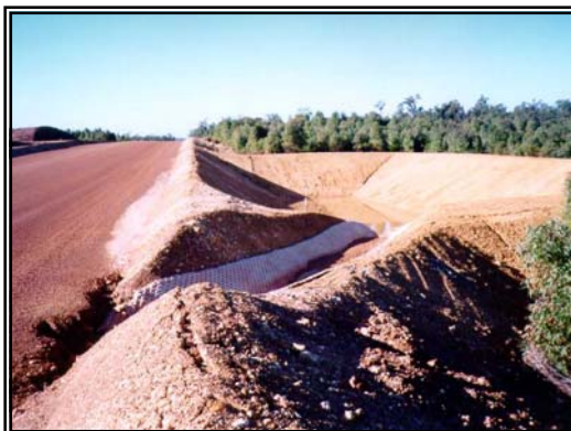
Figure 7.1 Drainage is captured and prevented from entering uninfested areas
