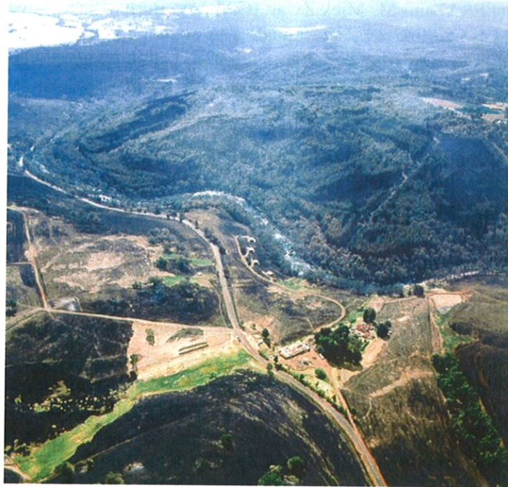
Figure 1. View NW from the Brockman Highway across the Blackwood River in early January 2004. Low lying areas still carried green grass at the time of the fire, while upland pastures were fully cured. The extent of crown damage in pine plantation north of the river varies from minor crown scorch through to complete defoliation. Buildings are on Loc. 6361.
