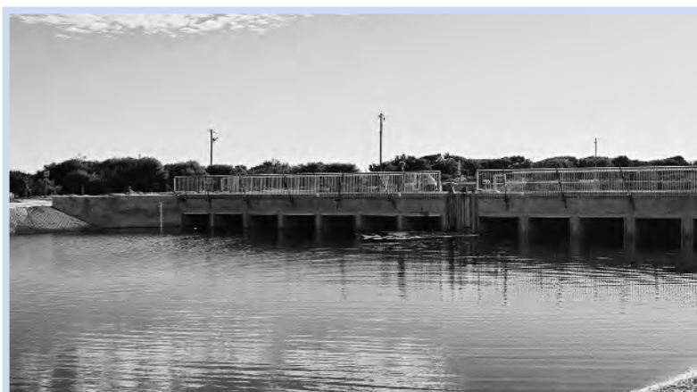
Floodgates on the Vasse Estuary replaced in 2004
