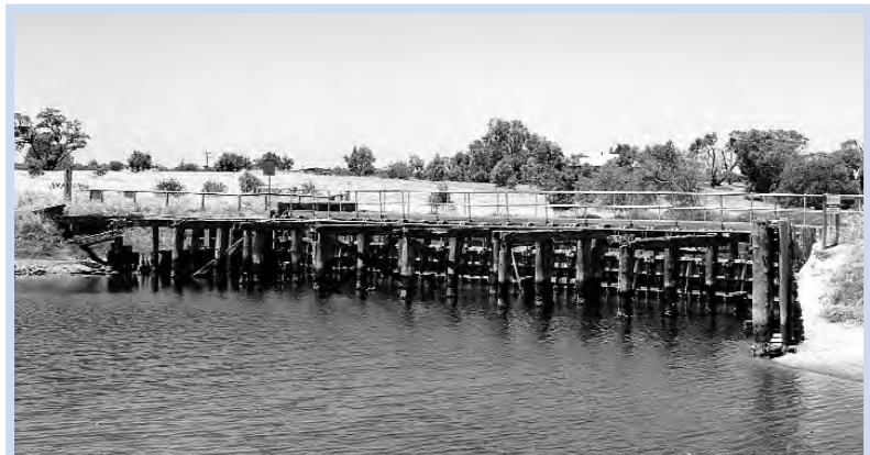
Floodgates on the Vasse Estuary
