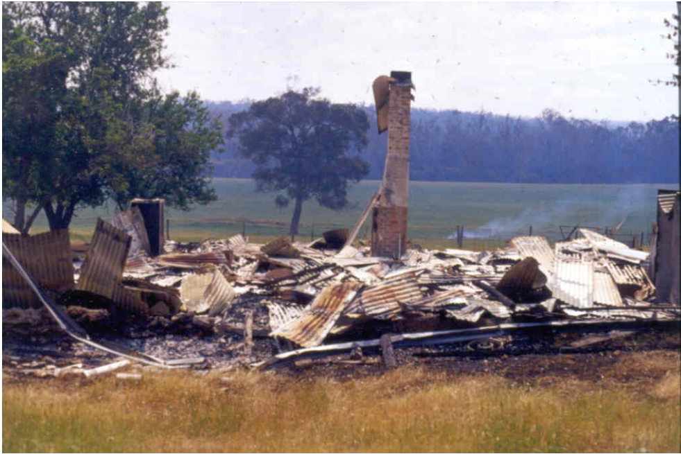
Figure 16. East side of the Hay River on Loc. 1899, showing the remains of the wood and iron house burnt on 15 November 2002. The photograph is looking west back towards the river. The grass surrounding the house was uncured at the time of the fire.
