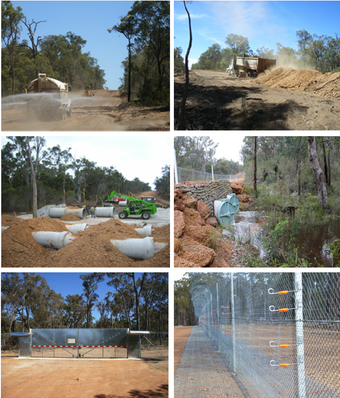
Figure 32. Selected images of design elements of the Perup Sanctuary infrastructure under construction including a & b) 12 m fence clearing and gravel road base foundation, c) culvert and pipe construction for drainage, d) detail of drain, e) vehicle access gate, f) detail of fence
