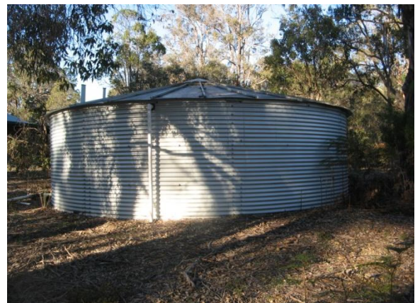
Figure 9: Current Rainwater Tank (Photo: Elise Pinto, 2011)
