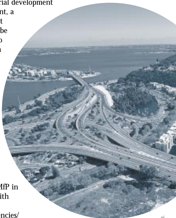
Aerial view of the freeway and Narrows Bridge, looking towards South Perth.
