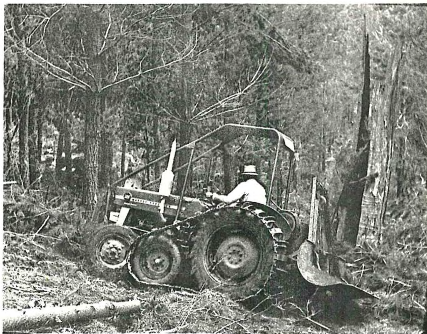
FIGURE 2. An M.P. 35 Tractor and half tracks turning on a 23° slope.
