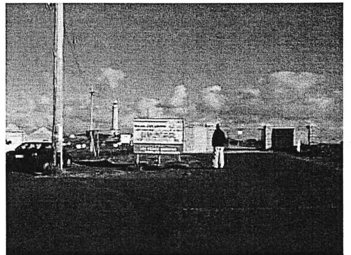
Existing entry gates to lightstation
