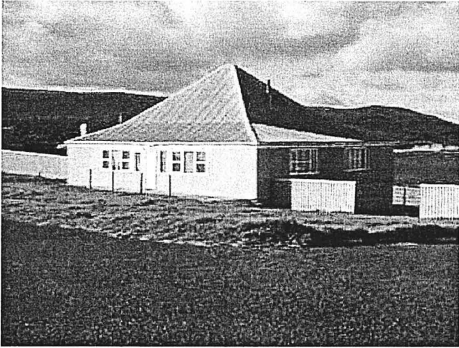
Lighthouse Keeper's Cottage
