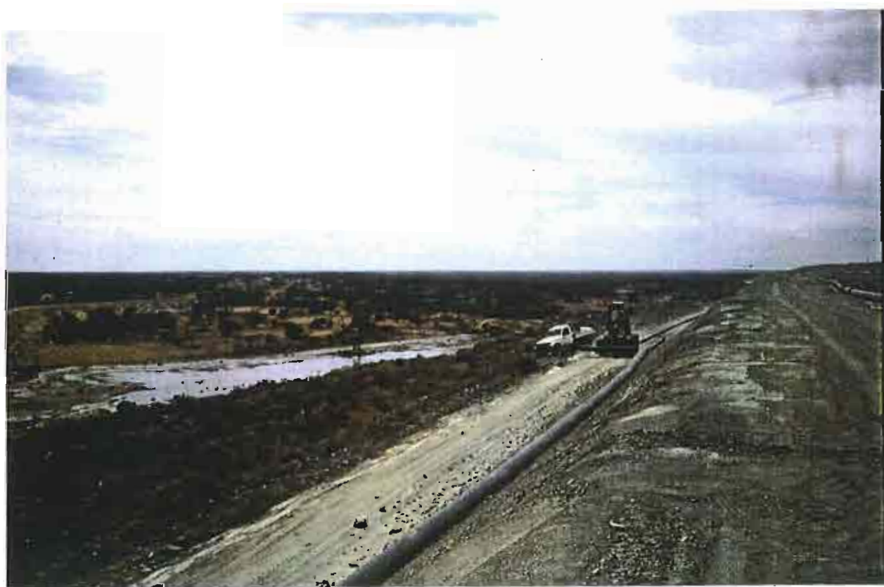
Plate 2b Big Bell Photo of leakage from the tailing facility taken from the crest of the embankment.
