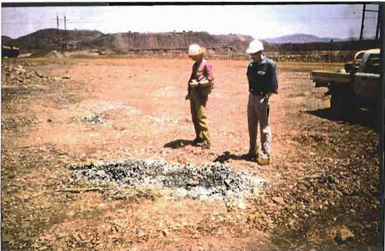
Plate 1b Mt Whaleback "Burn through" of cover material placed over reactive McRae Shale unit materials.
