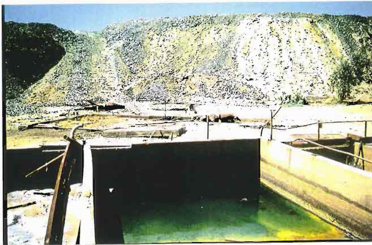
Plate 8a Nepean Intermediate processing facilities below waste rock dump. pH of standing water is 4.3.
