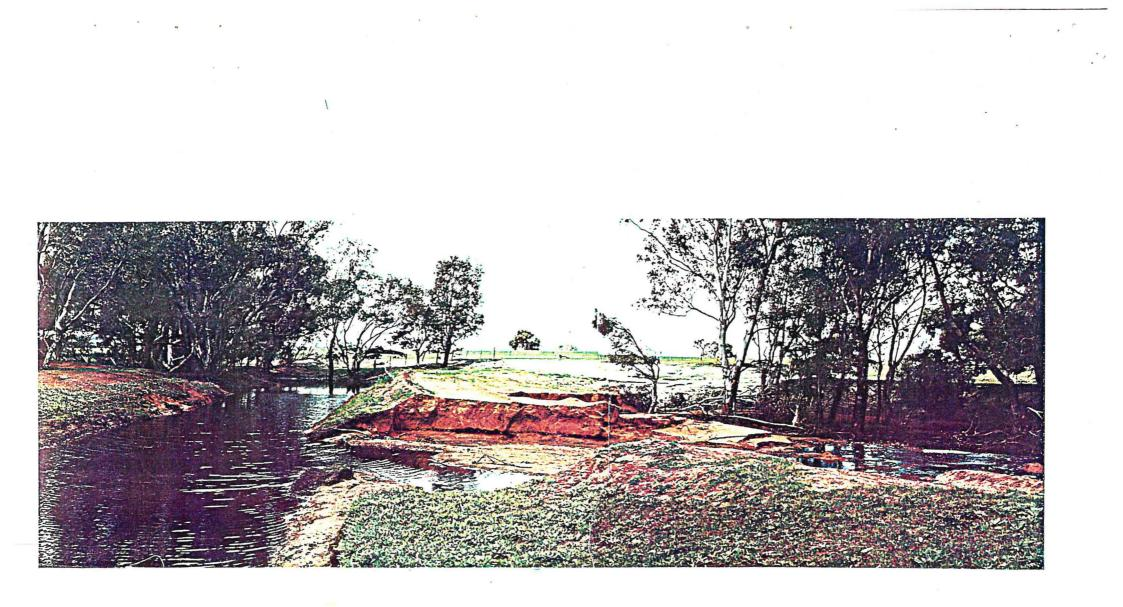
PLATE I - Taken 4/9/86 approx. 2-3 weeks after plug breached - initial flood flow ceased - had been 0.50 m higher. Flow across top of plug rapid and approx. 3.00 m wide x 5 mm deep.
