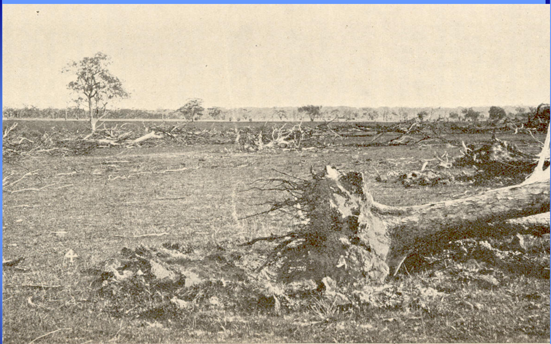
Clearing land by the "Forest Devil" on the Great Southern Railway.
