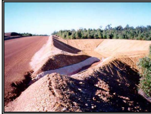
Figure 7. Drainage is captured and prevented from entering unfested areas
