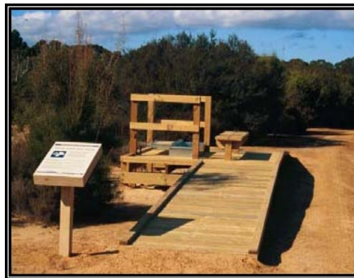
Figure 9. Simple boot cleaning station
