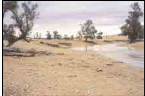
Figure 11.1. The impact of an over-enthusiastic contractor. This bank was meant to be only slightly battered, and the groynes should have been on the toe of the bank, protruding into the base flow.
