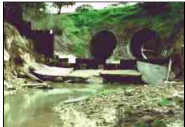
Figure 11. A railway crossing over Fells Creek, Gippsland, Vic, being threatened by erosion of the channel bed. Note the attempts to protect the structure.
