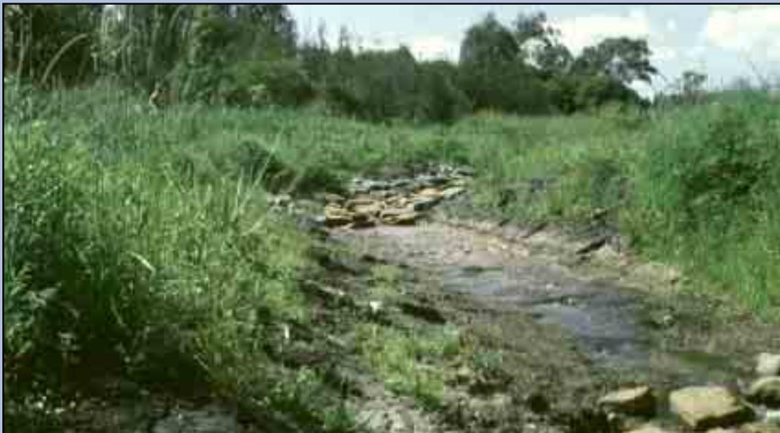
Figure 8. Artificial riffles constructed in a small stream in Brisbane by the Brisbane City Council.
