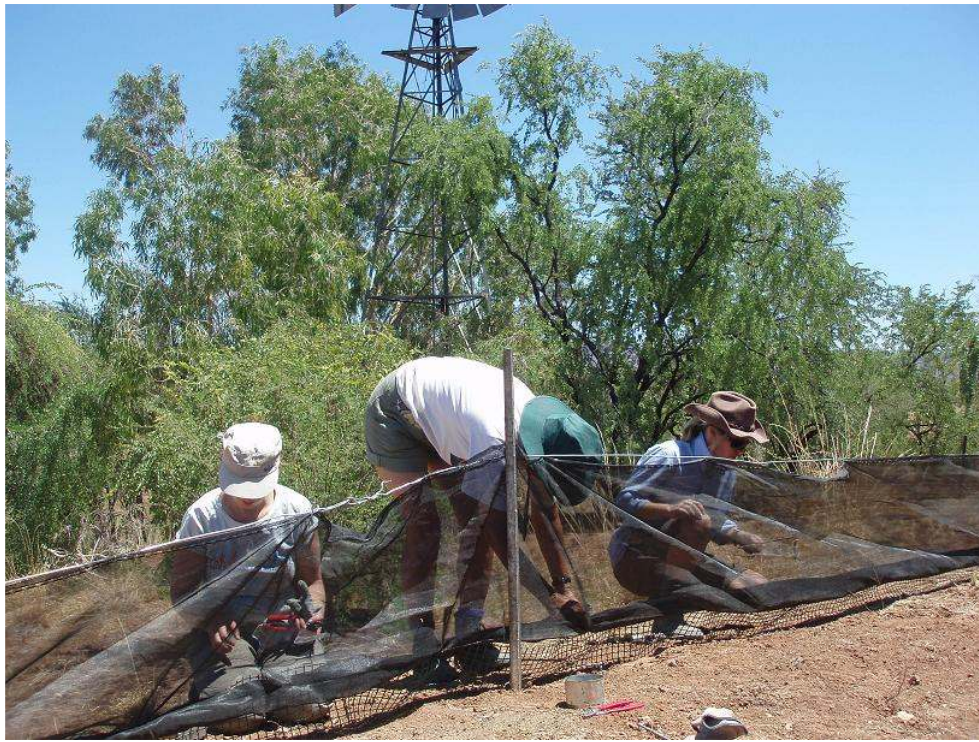
Volunteers inserting 25mm square mesh along the bottom of the fence as wildlife friendly gates.
