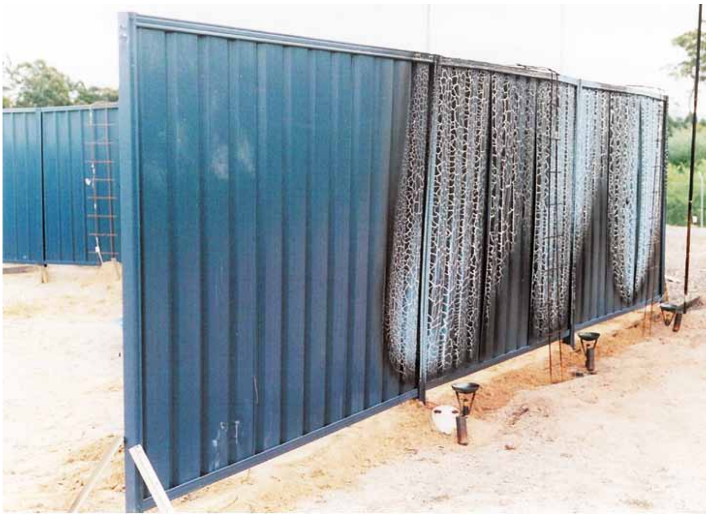
▲ A steel fence after testing at the Mogo site.
