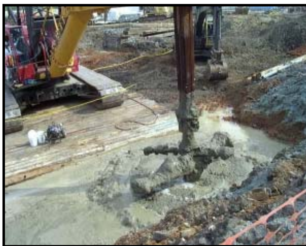
Figure 1 Deep soil mixing in peaty soils
