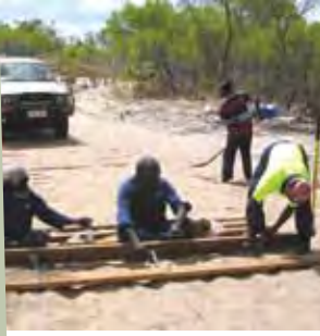
Boardwalk construction, NT (Photo: Anindilyakwa Land and Sea Rangers and DSEWPaC)
