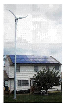
**FIGURE 3.3** Small wind turbine, shown near home with rooftop photovoltaic panels installed. Source: Courtesy of National Renewable Energy Laboratory. Electricity from Renewable Resources: Status, Prospects, and Impediments http://www.nap.edu/catalog/12619.html
