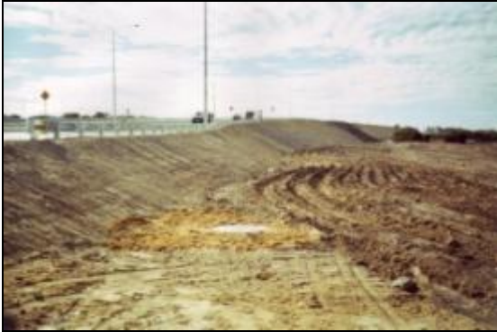
Batter banks before soil stabilisation with spray on Erosionex.
