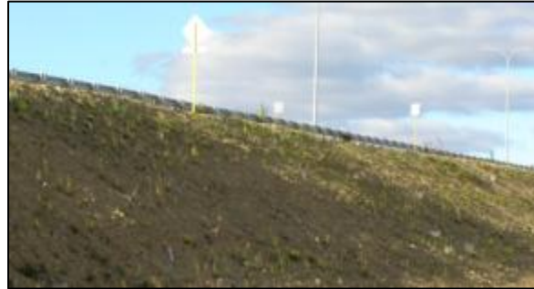
Germination of seeds on batter banks after application of Erosionex stabiliser.
