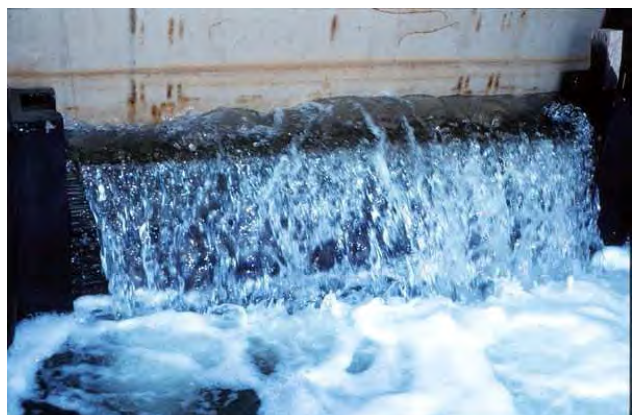
Photo 36: Leakage of seawater through Vasse estuary floodgates at high tide (16May1999).
