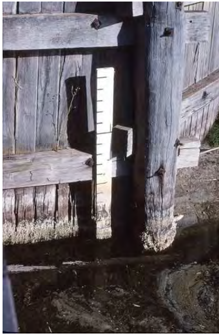
Photo 37: Former Water Corporation Vasse estuary gauge board at floodgates (25Jan1998).
