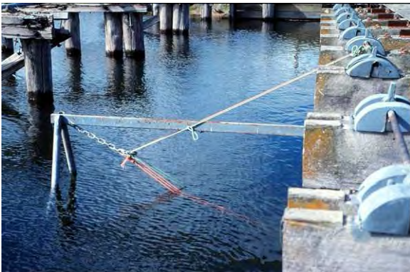
Photo 33: Vasse estuary floodgate temporary winch setup (16May1999).
