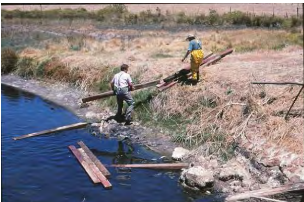
Photo 35: Manual removal of Wonnerup estuary floodgate stopboards for fish release (18Jan1998).
