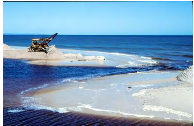
Photo 40: Water Corporation contractors closing Wonnerup Inlet sand bar (22Oct1999).
