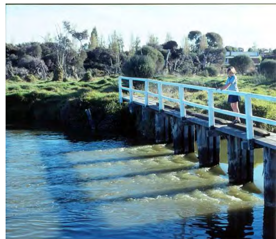
Photo 42: Flow through recently-opened 'check structure' on Vasse River at Butter Factory Folk Museum (03Apr1998).
