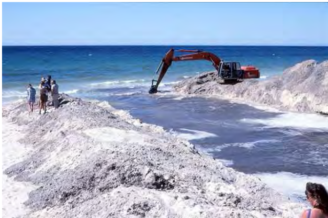
Photo 39: Water Corporation contractor opening Wonnerup Inlet sand bar (02Jan1998).
