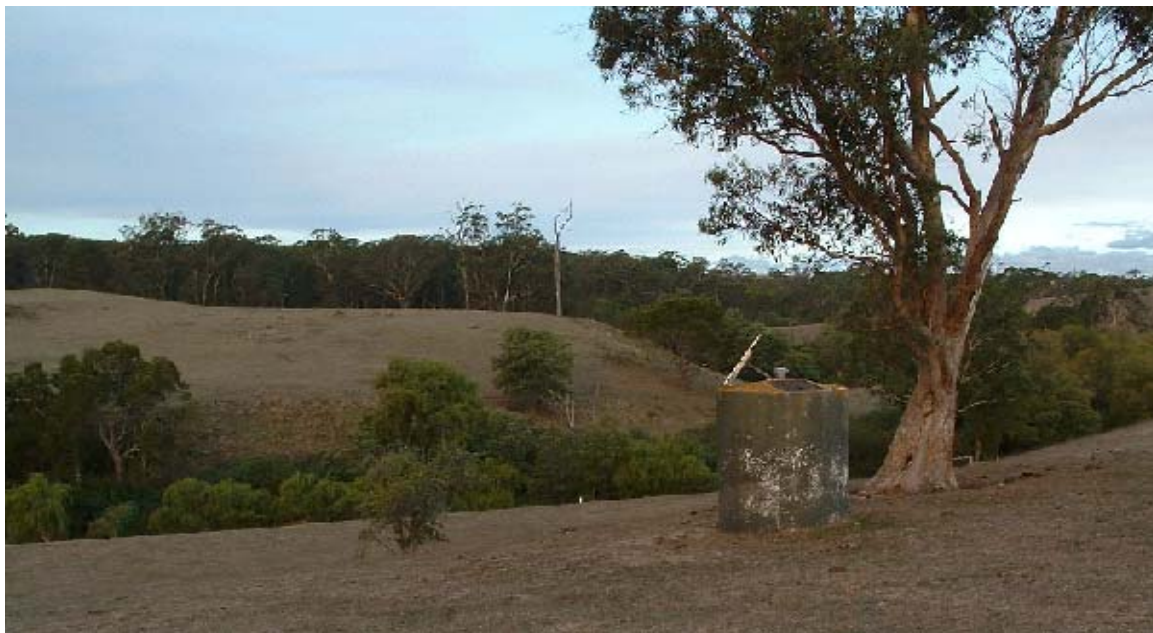
Figure 1. The gauging station for the Merrimans Creek at Stradbroke West.
