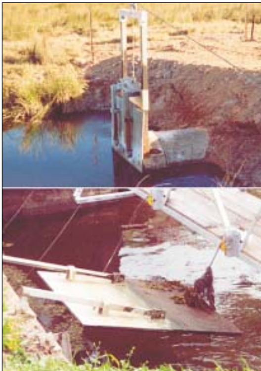
Figure 23. Vertical winch gates (above) and horizontal winch gates (below). Both are opened via a cable and pulley system attached to a stationary winch on the bank. (Photos: Rob Lloyd and Alan Cibilic)
