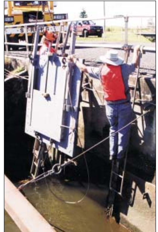
Figure 56. Installing sluice gates on the Empire Vale drainage system. Selecting drain system management methods should be based on clear objectives and a sound understanding of the key features of the drainage system (see pg 14). The concerns of all stakeholders need to be considered. (Photo: Jon Woodworth)
