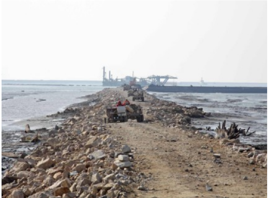
New seawall construction © A Boyle
