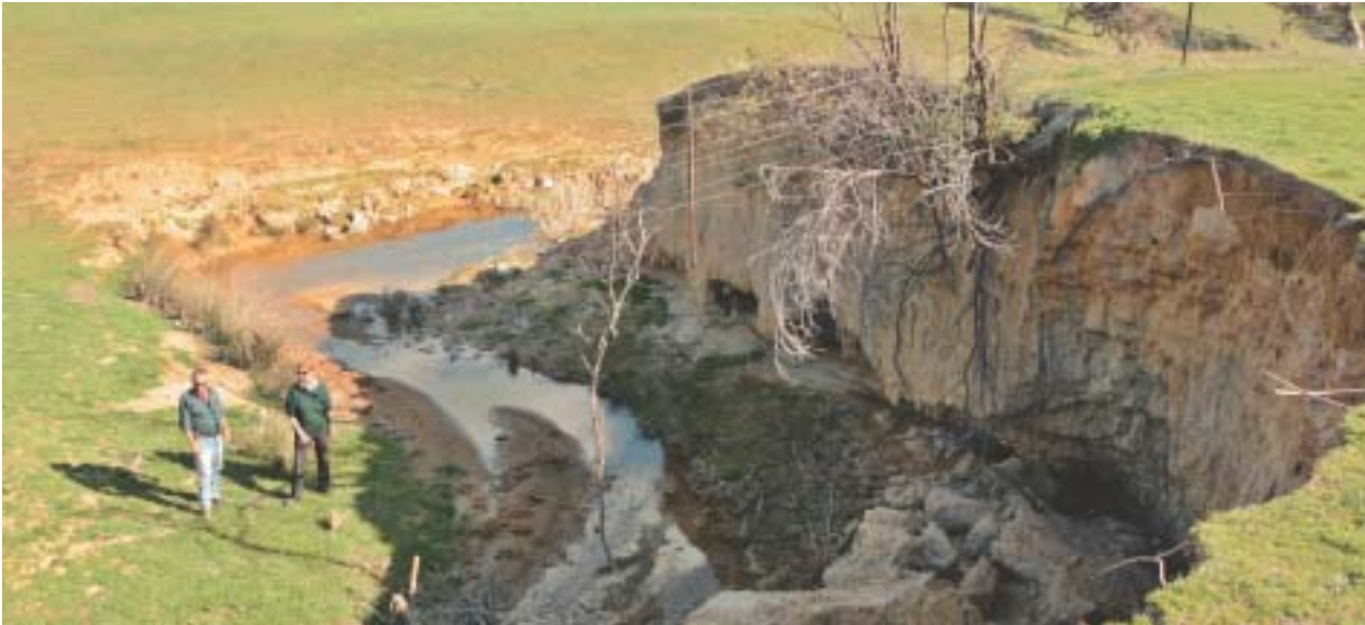
A mass failure event resulting in large scale streambank erosion, NSW. Photo Gary Caitcheon.
