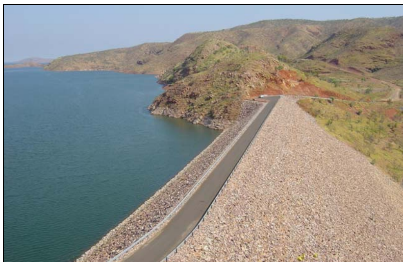
Lake Argyle dam wall. Water from the dam is used for irrigation in the lower Ord around Kununurra and also for hydro electricity for Kununurra township and Argyle Diamond Mine.
