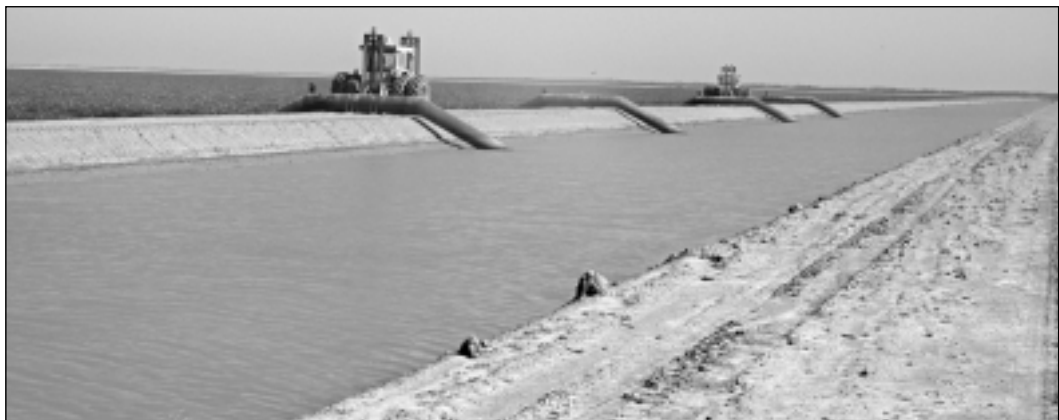
Irrigation with over the bank siphons
