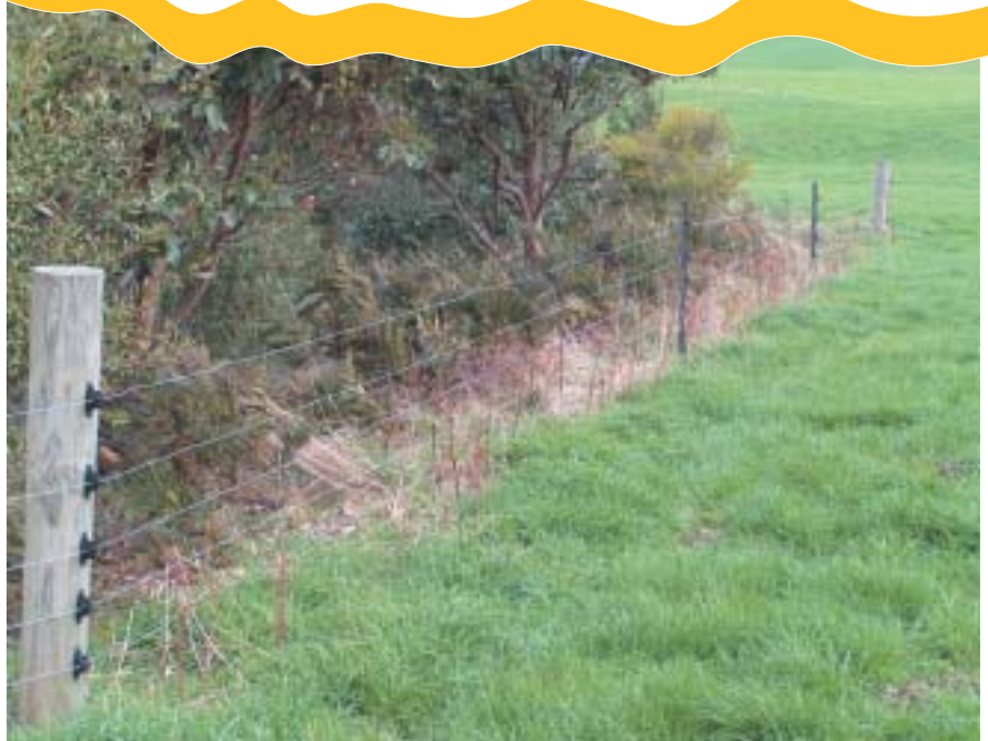
Electric fence built using a combination of posts and pickets. Photo Jenny O'Sullivan.
