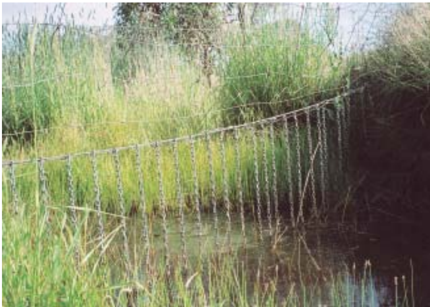
Electrified chain floodgate.
