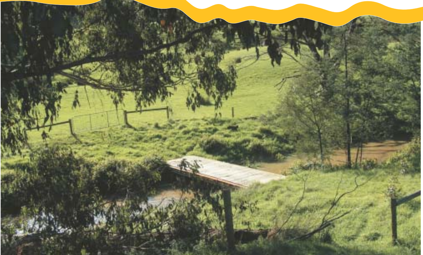
Well-sited crossing made from a truck tray. Note the gates at either end of the crossing. Photo Jenny O'Sullivan.
