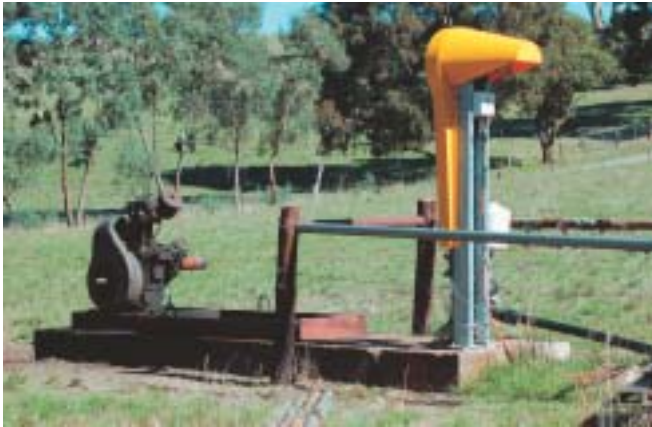
Solar powered pump with back up petrol pump. Solar panel shown above right. Photos Roger Charlton.
