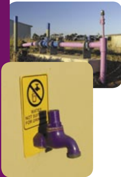
Figure 4 Example of lilac colouring of pipe and tap required for recycled water use in agricultural and urban areas
