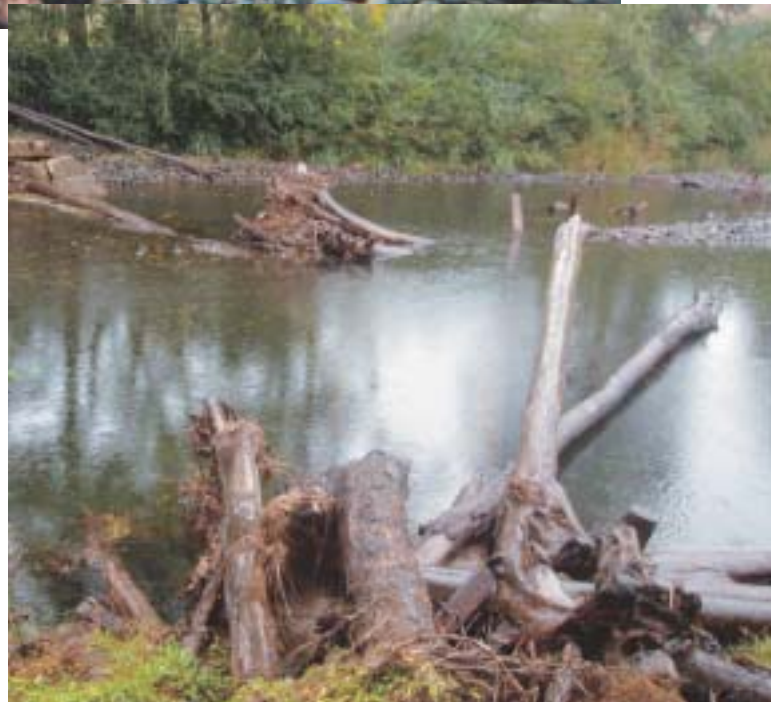
Photo 36. “Failed” cross-spanning log bed control structure on the Williams River. This structure failed when one of the key abutting logs in the centre of the channel was removed in a flood. Note, the abutting log jam in the foreground is still functioning and most of the logs in the channel centre are still providing good habitat value. This structure has, therefore, only failed in an engineering sense.
