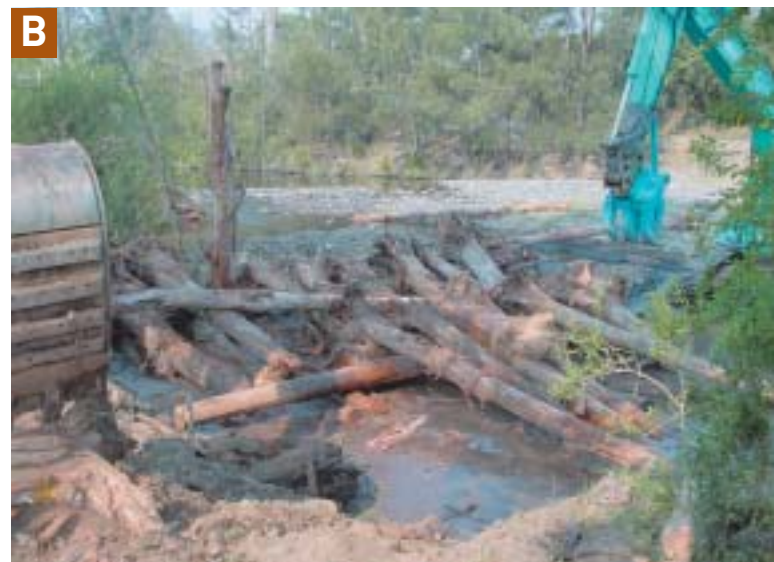
Figure 22. Construction sequence for a standard deflector jam. (A) Excavated pad ready to begin construction of a large deflector jam. (B and C) Upper layers of the longitudinal logs being arranged on structure. (D) Completed structure. Photos T. Abbe.
