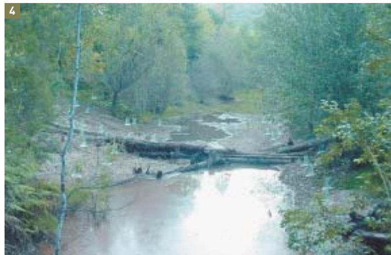
4. Completed structure looking upstream.
