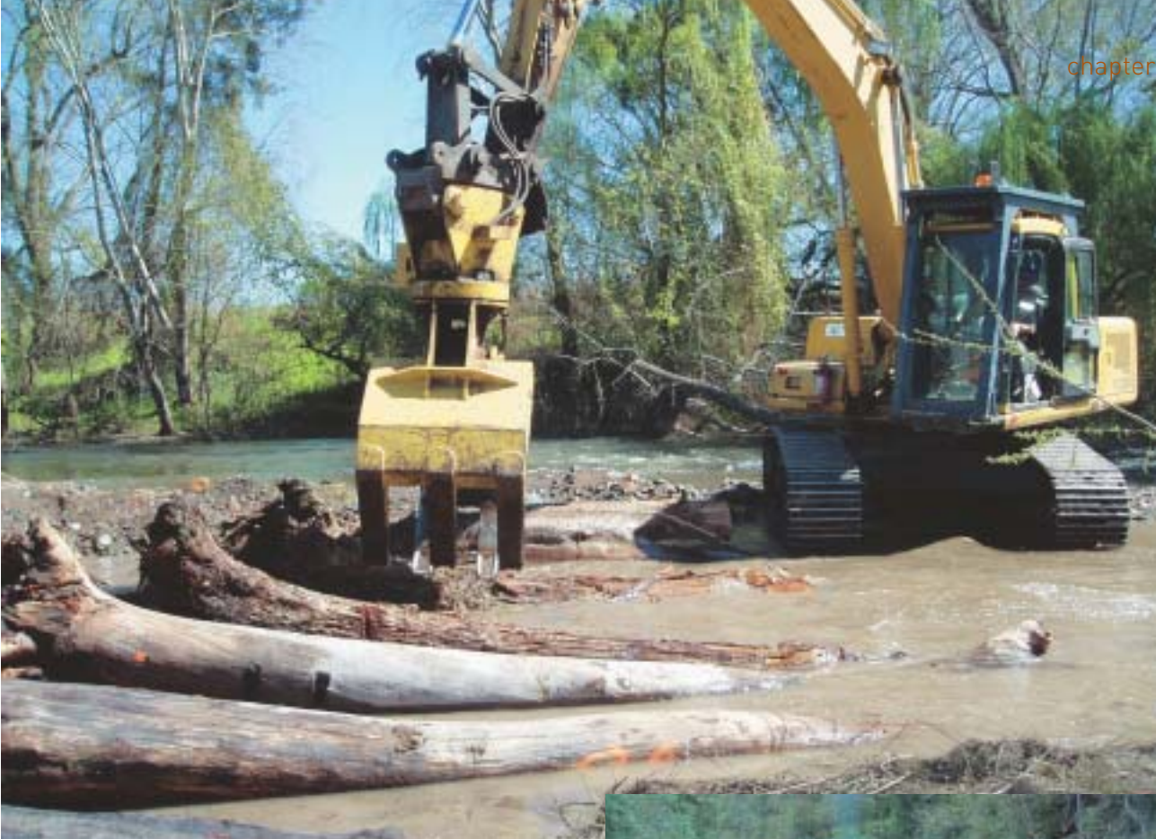
Photo 38. A universally rotating log grab makes log placement a much easier and more efficient process.
