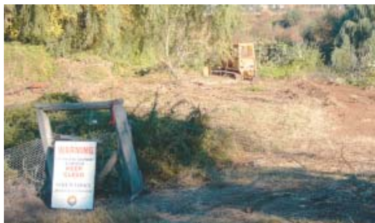
Photo 43. Warning signs should be erected at your project site to indicate the boundaries of the project area.
