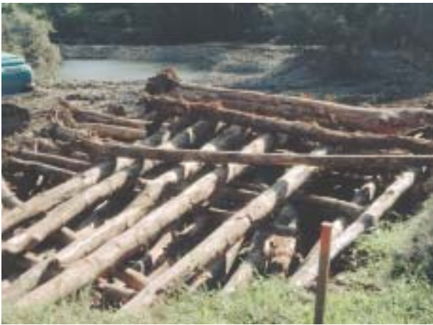
Photo 2. Bank deflector jam under construction — Williams River, NSW.
