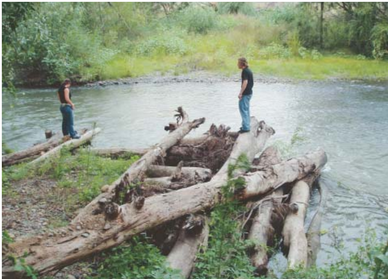
Photo 9. Constructed log jam — Hunter River, NSW.
