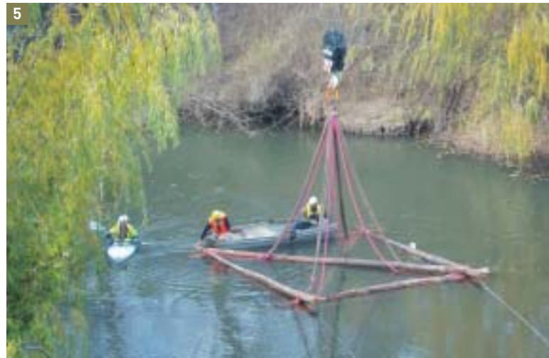
5. Fish hotel being positioned in pool 1.
