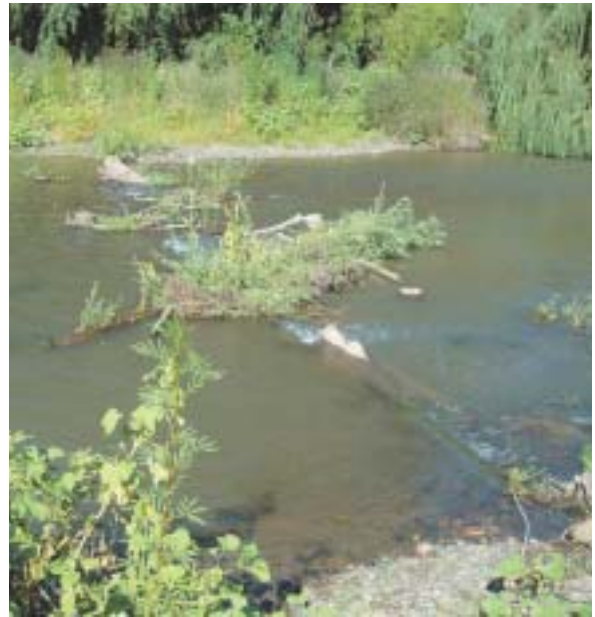
Figure 5. This constructed deflector jam (DFJ) extending into the channel in the Williams River caused scalloping of the edge of the gravel bar across the channel, enhancing the surface area for lateral hydrological exchange, represented by arrows in the schematic diagram.
