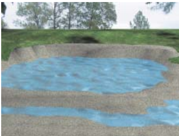
Step 1. Excavate pad and construct check dam to isolate pad from river channel.
