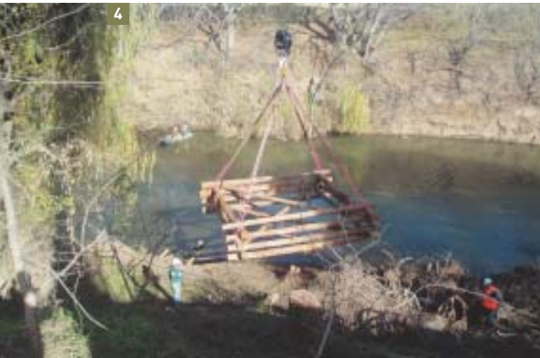
4. Fish hotel being lowered into pool 1.
