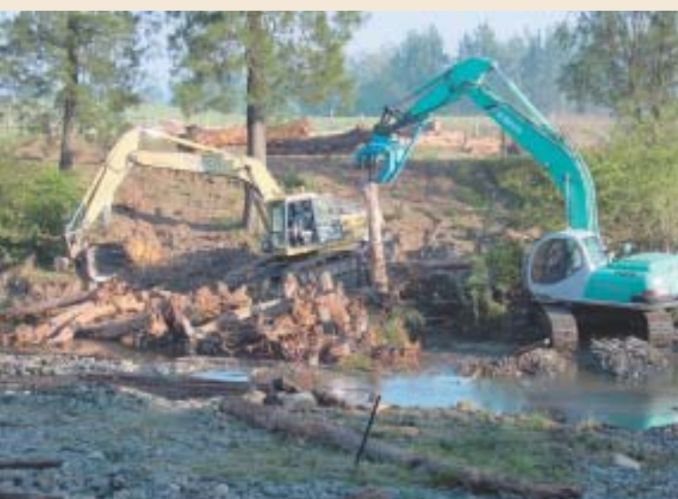
Photo 37. DFJ construction in full swing — Williams River, NSW.
