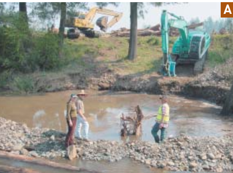
Figure 22. Construction sequence for a standard deflector jam. (A) Excavated pad ready to begin construction of a large deflector jam. (B and C) Upper layers of the longitudinal logs being arranged on structure. (D) Completed structure. Photos T. Abbe.
