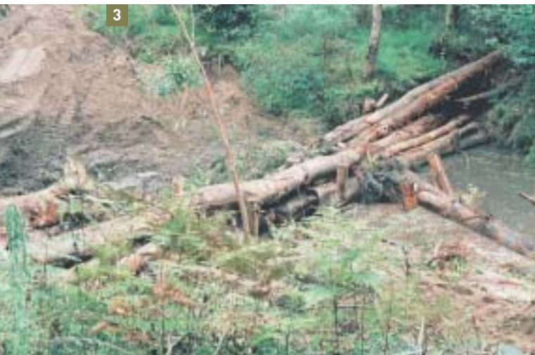
3. Cross channel spanning structure with bank abutments nearing completion.
