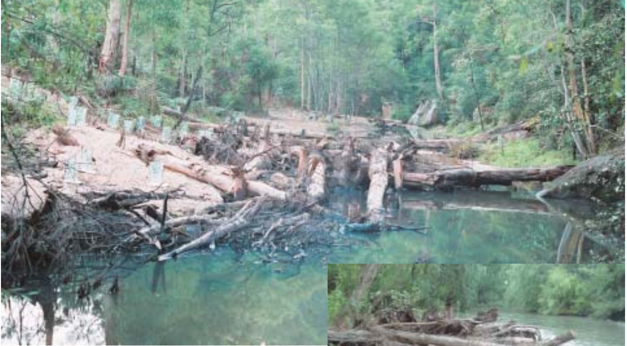
Photo 12 (above). Constructed log jams — Stockyard Creek, Hunter Valley, NSW.
