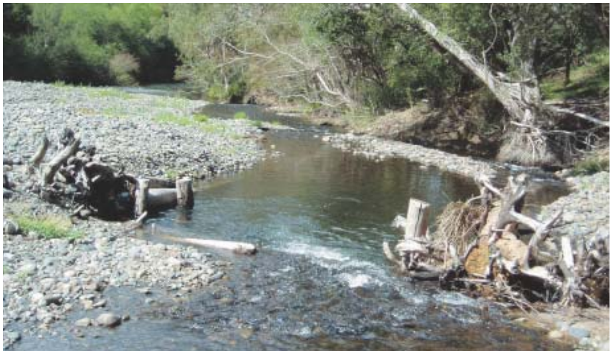
Photo 7 (below). Constructed hyporheic jam (i.e. log step with paired abutment jams) — Williams River, NSW.
