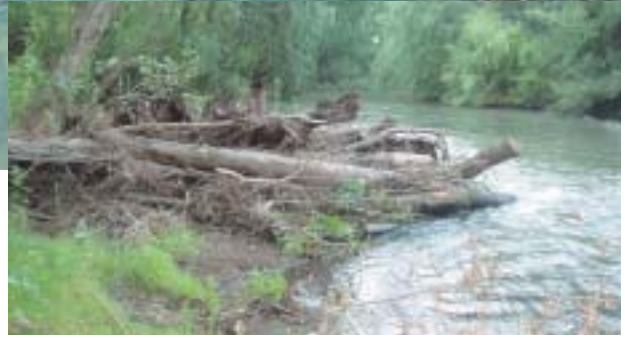
Photo 12 (above). Constructed log jams — Stockyard Creek, Hunter Valley, NSW.
