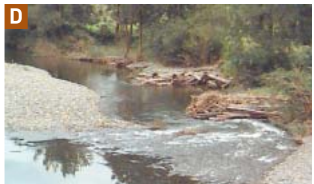
Figure 13. (A) Upper section of Munni test reach at the commencement of construction of DFJ1. Note a 4 m high actively eroding bank was located to the right of the tractor; (B) DFJ 1 and 2 at the completion of construction; (C) Same view in flood ( 270 \text{ m}^3 \text{ sec}^{-1} , 7/05/01) at about 1 m below peak stage; (D) DFJ 1 and 2 after the second major flood since construction — note the aggraded bar upstream of first structure and the increased scour around the two structures. The riffle crest in the foreground was raised, we presume due to backwater effects associated with the structures.
