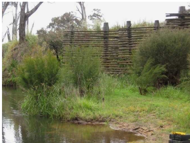
Site 2-2: wooden barrier to deflect high flows and reduce bank erosion along main channel
