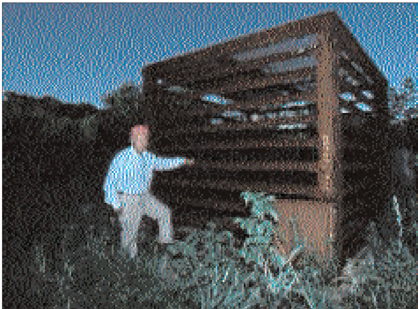
This protective cage at the Neda Mine in Dodge County, Wisconsin, ensures human safety while also protecting one of North America's largest hibernating bat populations. It cost less than alternative methods of closure and was built through collaboration of the Wisconsin Department of Natural Resources, the University of Wisconsin at Milwaukee, and the Friends of the Neda Mine—a private group led by Bat Conservation International Chairman Emeritus Verne (pictured) and Marion Read.
