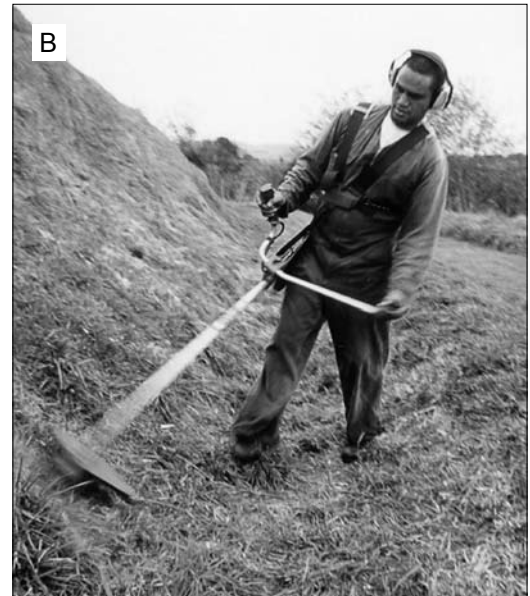
Figure 32. The bad and the good in grass-cover management. A. Ride-on mowers often create scalping where there is a rise in the ground surface. B. Banks should be cut with a weed-eater.
