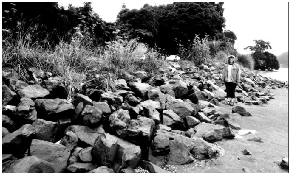
Figure 8. Rip-rap sea wall protecting areas of the site of Tokitoki, Ohiwa Harbour.
