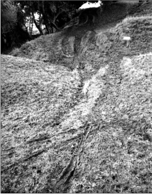
Figure 5. Typical branching tracks in summer (left) and winter (above) on One Tree Hill. The multiple tracks are formed because people prefer to walk on a grassed surface rather than a muddy or dusty one. The solution is to limit visiting, or to re-route and re-design the track so that people are comfortable walking on it. Photographs: Dianne Harlow.
