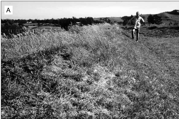
Figure 32. The bad and the good in grass-cover management. A. Ride-on mowers often create scalping where there is a rise in the ground surface. B. Banks should be cut with a weed-eater.
