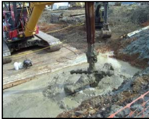
Figure 1 Deep soil mixing in peaty soils.
