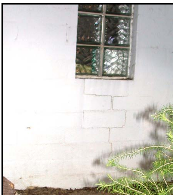
Figure 3. Cracks in external walls
